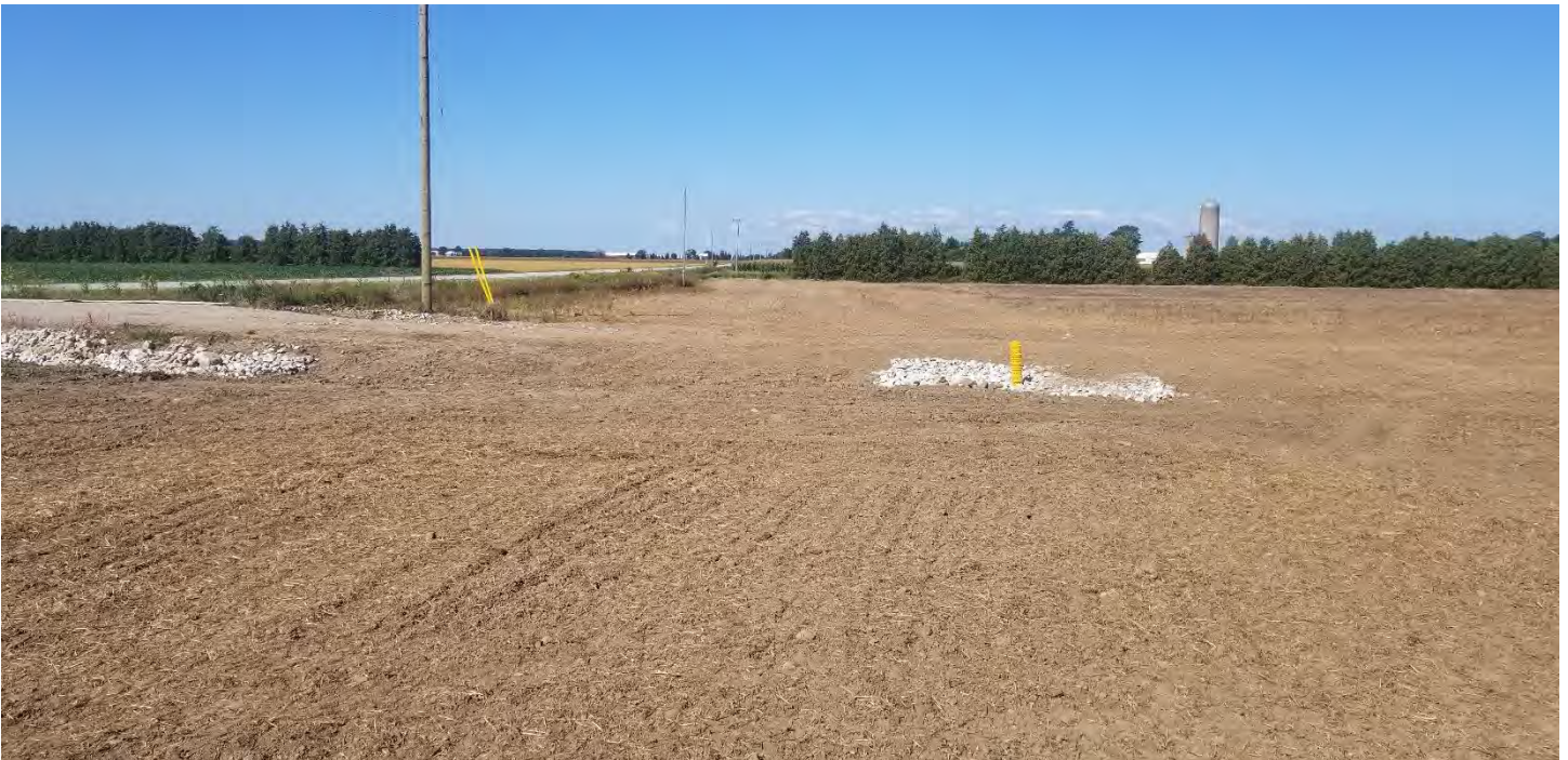
Photo of seeded low-level berm with the “upstream” hickenbottom, and rock chute (looking west)
