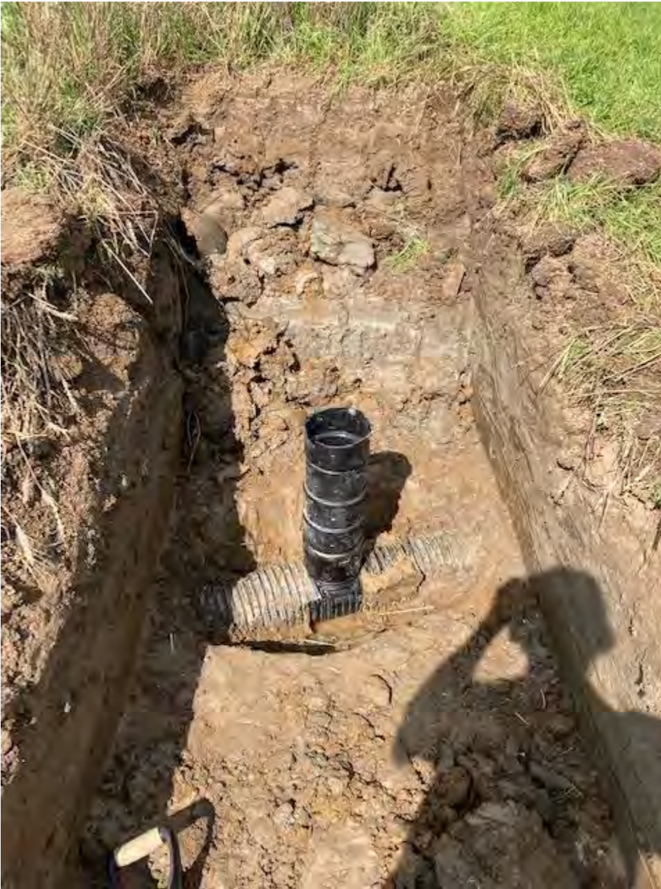
Photo of riser connection to tile
