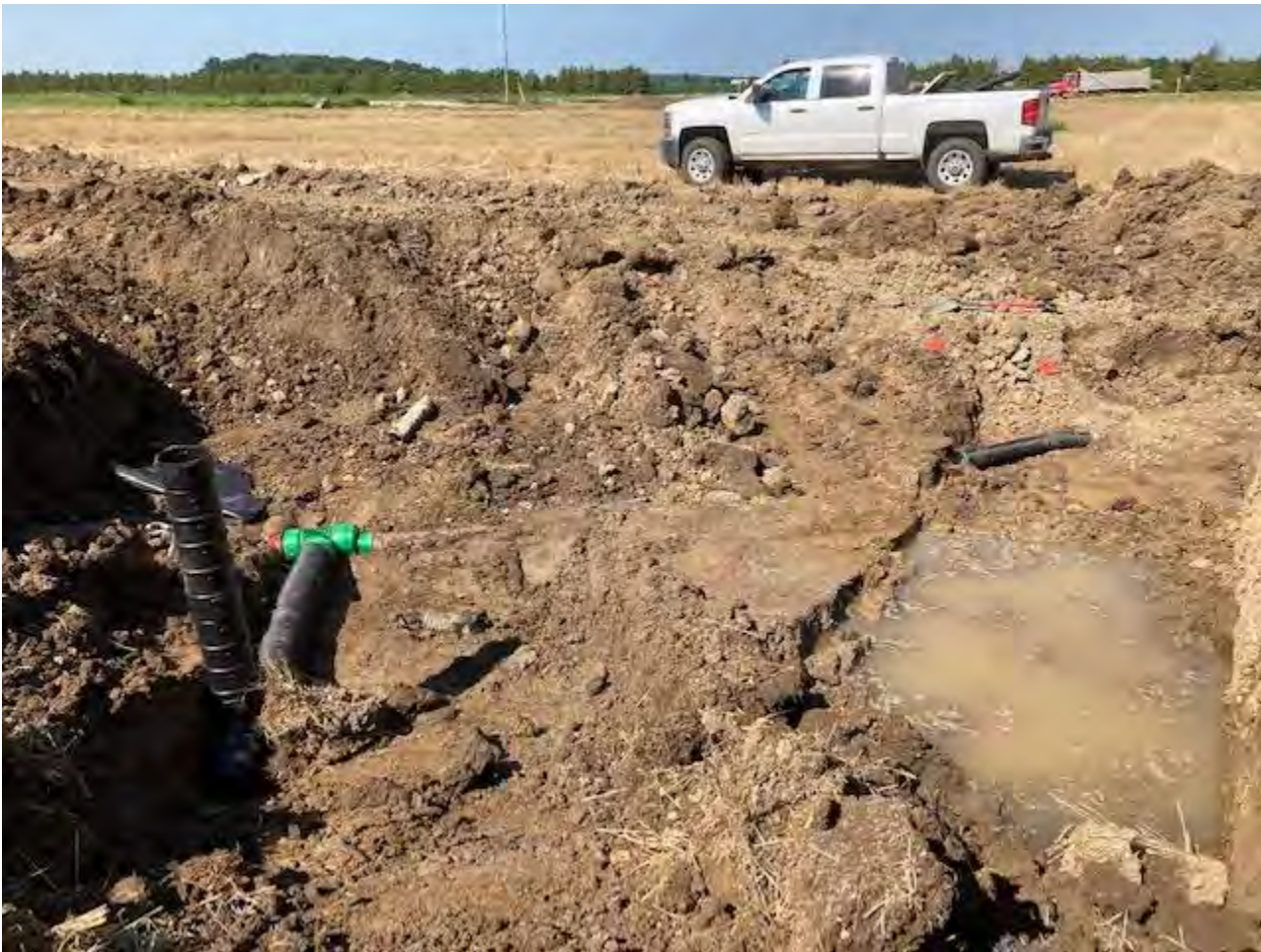
Attaching riser (hickenbottom) to existing tile
