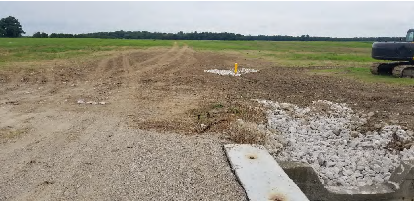
Photo of seeded low-level berm with the “upstream” hickenbottom, and rock chute (looking west)
