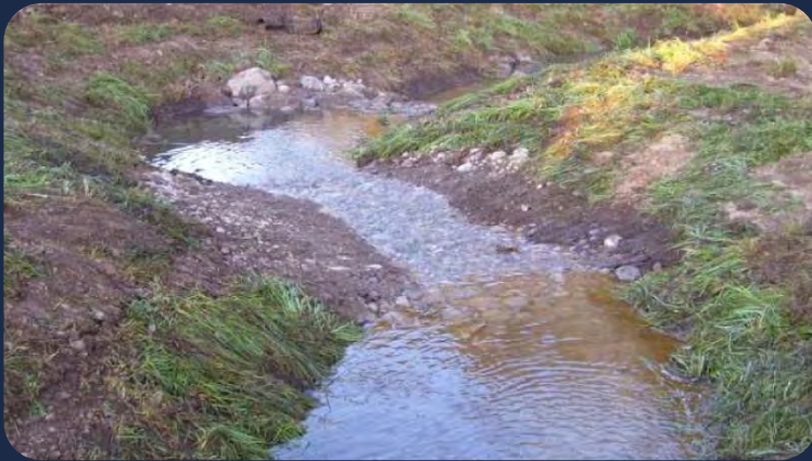
Riffles and Pools post-construction
