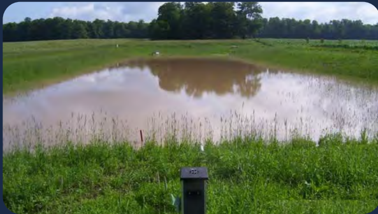
Wetland A with flow control box
